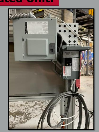
• All components are mounted on a portable aluminum extrusion frame allowing for modular positioning of each component. All electrical components are powered by a single 240v, 50 Amp power cord and subpanel.
